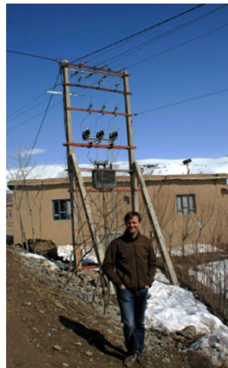
Electricity distribution system, installed by ESRA. Poles are made on-site from concrete because they would be too heavy to carry to the site.
